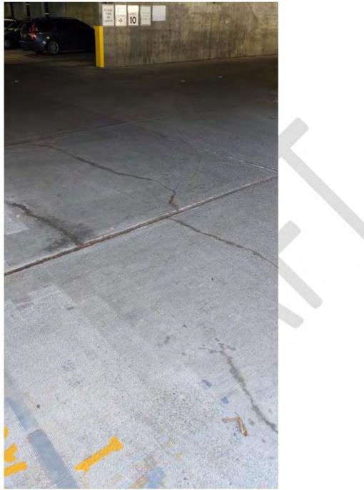
Figure 12 - Deck Cracking at North Entry
