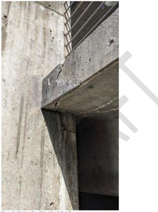
Figure 8 - Patch at East Side of South Exit Ramp
