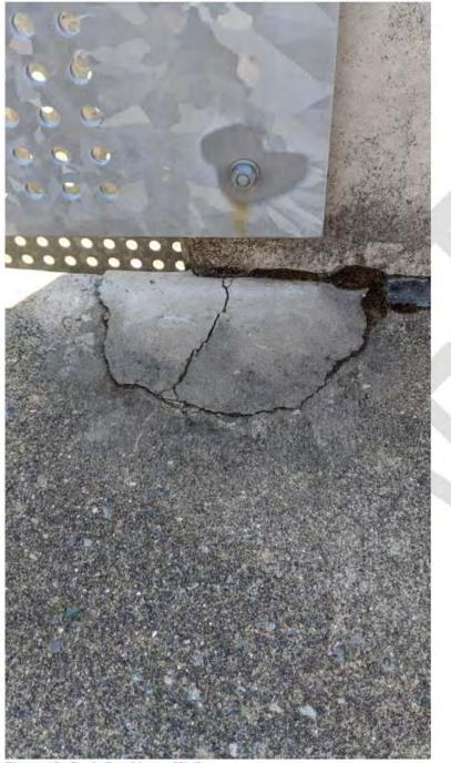
Figure 15 - Deck Cracking at Walls
