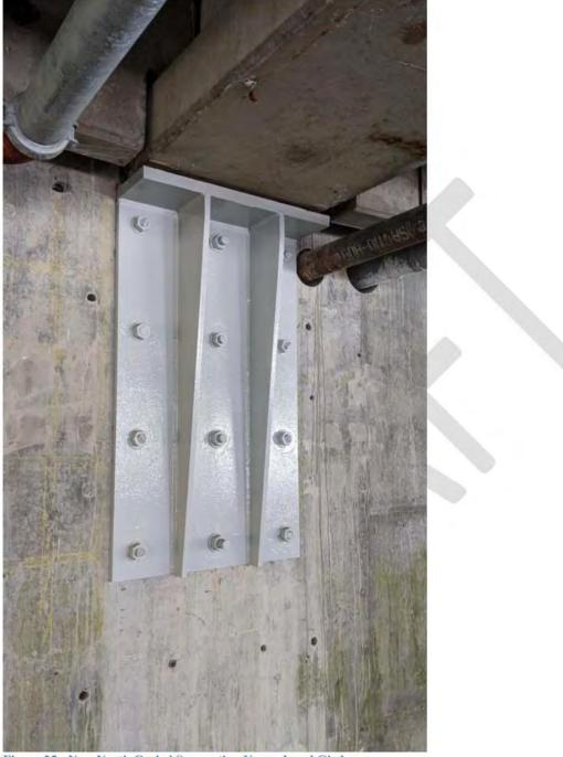
Figure 25 - New North Corbel Supporting Upper Level Girder
