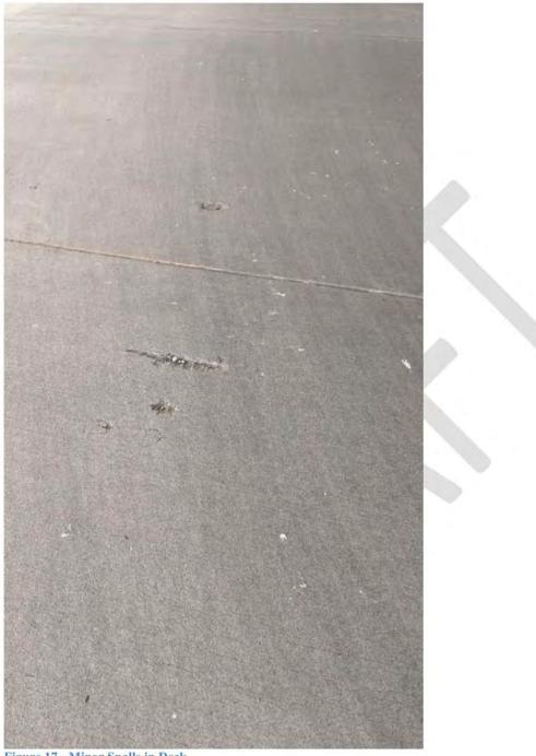
Figure 17 - Minor Spalls in Deck
