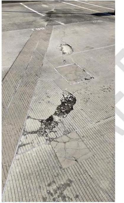
Figure 28 - Cracking, Spalling and Potholes in Upper Level Deck
