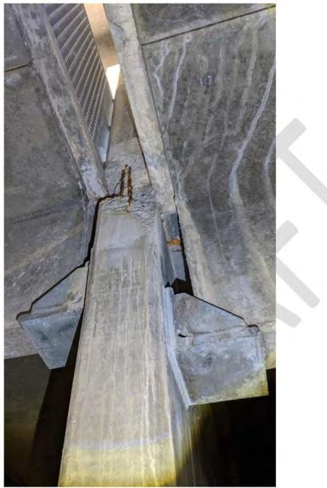
Figure 9 - Center Wall Spall (appears to have been patched and re-spalled)
