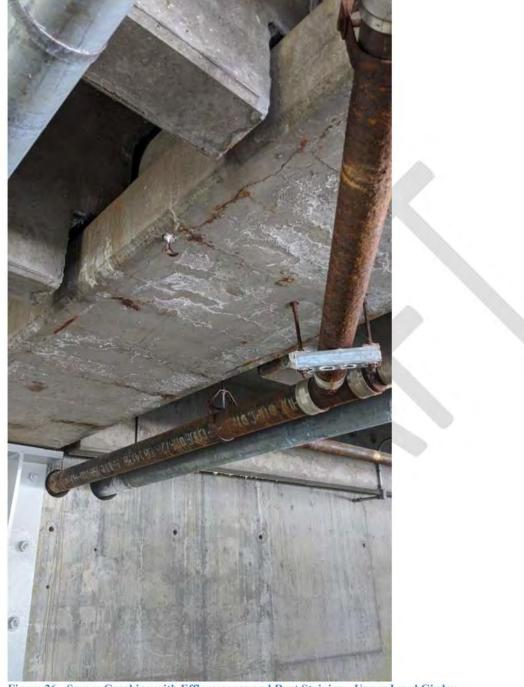
Figure 26 - Severe Cracking with Efflorescence and Rust Staining - Upper Level Girder
