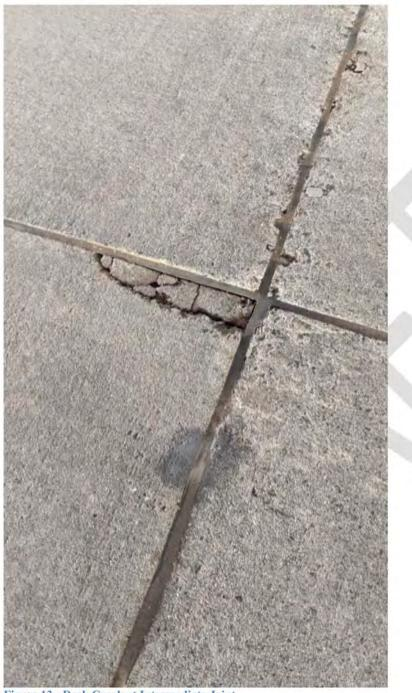
Figure 13 - Deck Crack at Intermediate Joint
