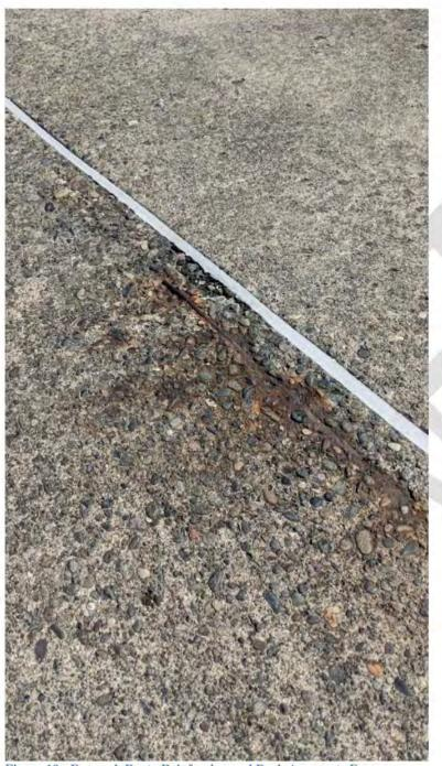
Figure 19 - Exposed, Rusty Reinforcing and Deck Aggregate Exposure
