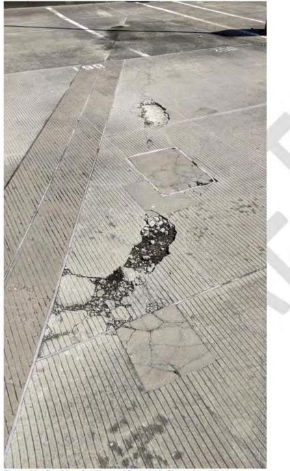
Figure 29 - Cracking, Spalling and Potholes in Upper Level Deck
