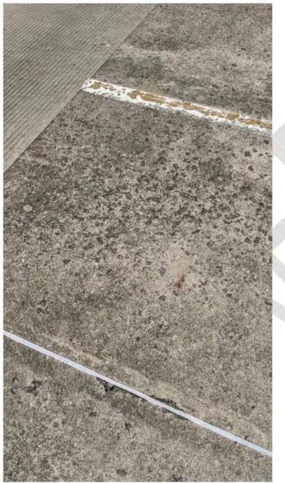
Figure 21 - Deck Aggregate Exposure
