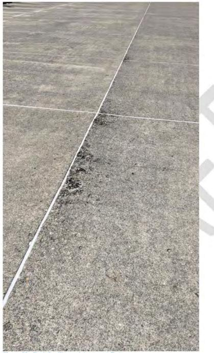
Figure 20 - Deck Spalling and Aggregate Exposure
