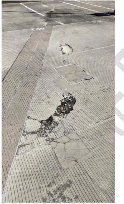
Figure 24 - Cracking, Spalling and Potholes in Upper Level Deck
