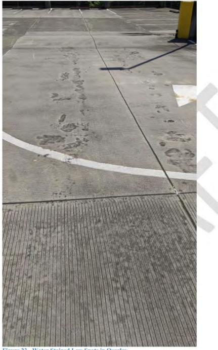
Figure 23 - Water Stained Low Spots in Overlay
